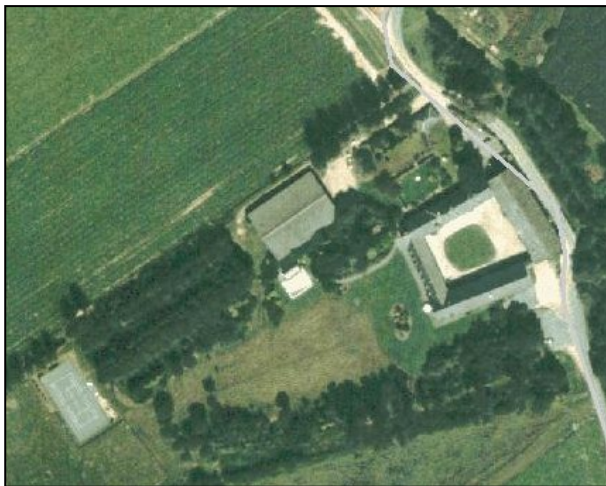
Figure 14: Aerial photography of 1997 (© RW)
